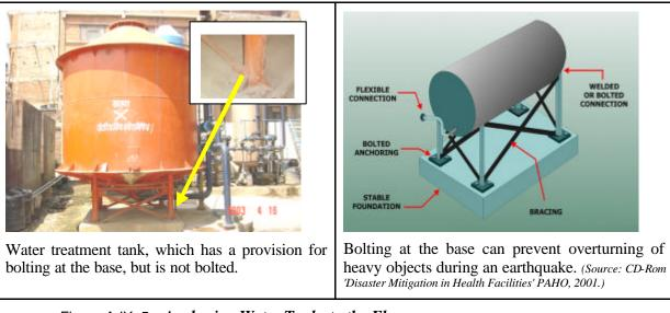
Figure A-IX. 5: Anchoring Water Tanks to the Floor.
